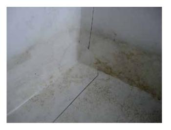
After two years lining the growing boxes, the MAPEPLAN T B lining proves perfectly undamaged and features no signs of piercing or deterioration either on the surface or along the main and detail welding.
