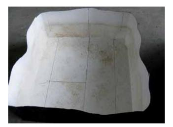
The root-resistant membrane must be placed inside the boxes according to a specific arrangement and must feature welding, T-joints and 4 corners.
