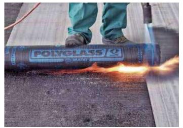
Membrane from Reoxthene line being torched on.
