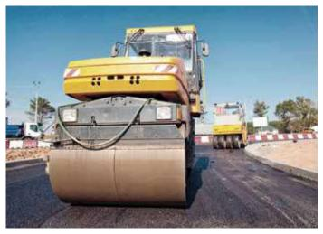
Compacting and finishing of the bituminous binder course.
